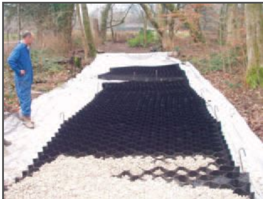
Geotextile Layed Out and Cellular Confinement System Pinned In Place
