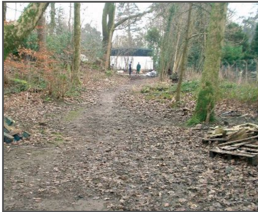
Area For Installation Is Cleared and Marked Out
